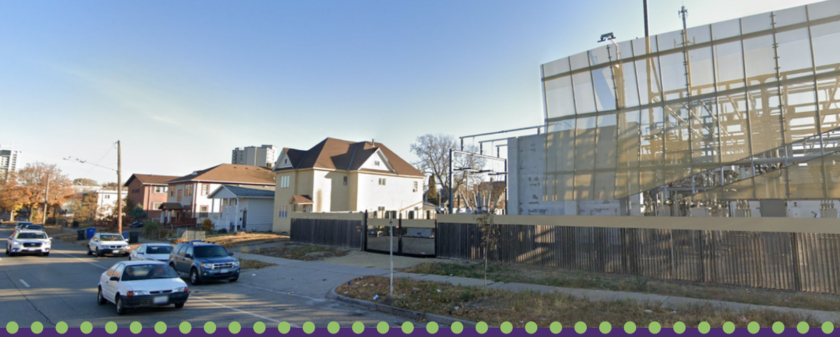
Xcel Energy's Midtown Substation in Phillips
