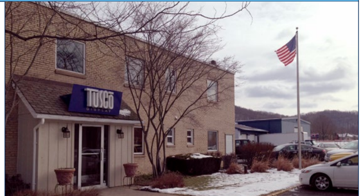
Figure 1: Tusco Display’s primary manufacturing facility in Gadenhnutten, Ohio is comprised of adjoining buildings constructed between 1946 to 1988, totaling 93,000 square feet. A 400-foot-deep well for a geothermal heat pump sits at the base of the flagpole.
