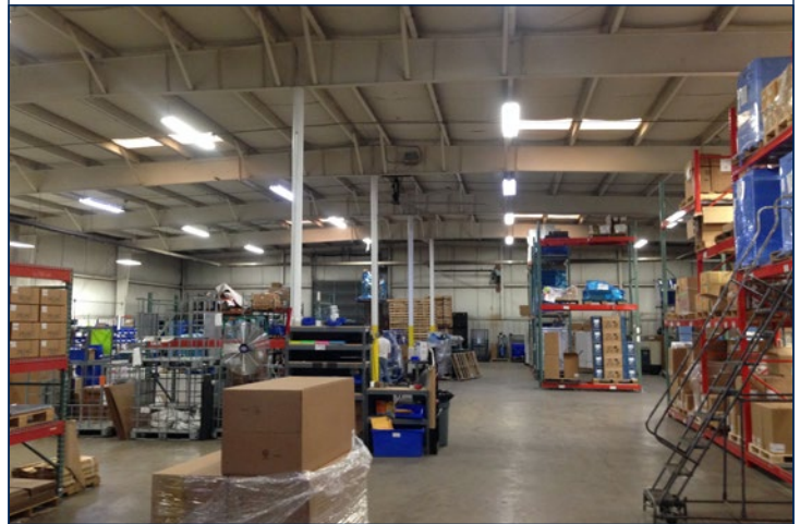
Figure 3: Tusco's 15,000-square-foot facility in New Philadelphia utilized on-bill finance to install T5 fixtures in 2013. Using company funds, an 18-foot-diameter overhead fan was also installed to better circulate indoor air.
