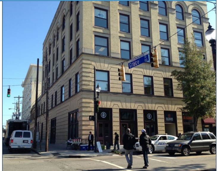
Figure 1: 272 North Front Street in Wilmington, NC
