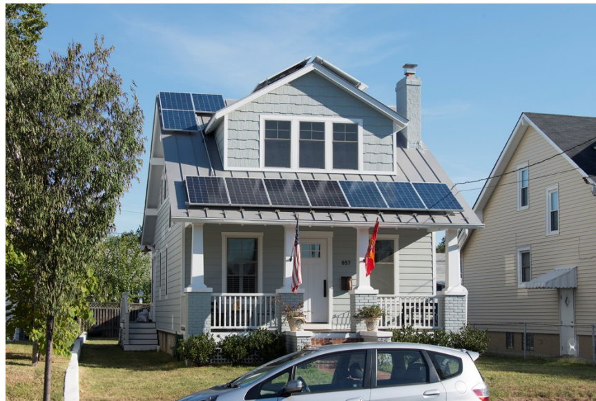
Figure 1: Single-Unit Detached. A dwelling that is designed for occupancy by one family. 11
