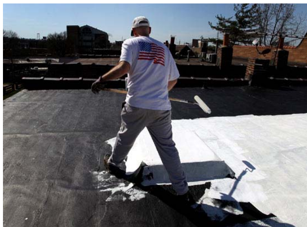
St. Louis volunteer coats a tar roof with reflective white coating.
